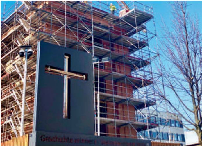
The construction site of the Garrison Church tower.
